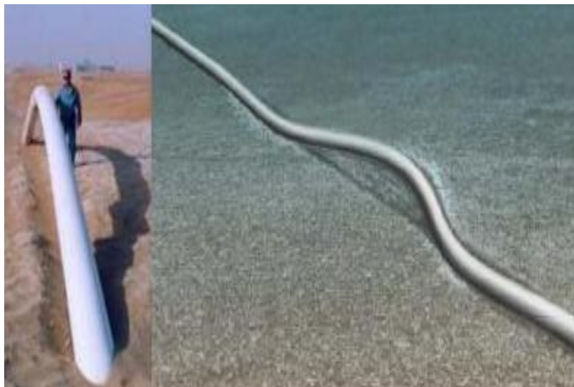
Figure III. 4 Dommages mécaniques (ondulation) [34].
