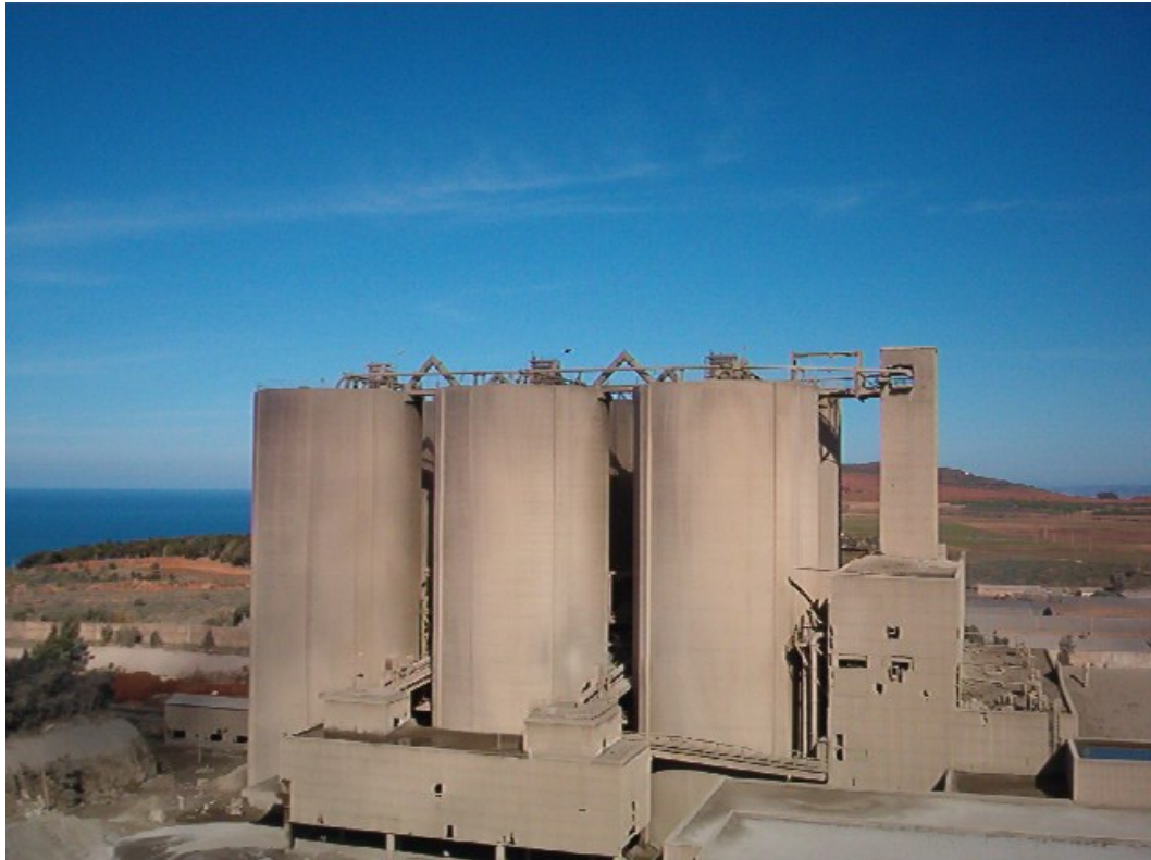
Figure 1.18 Silos de stockage
