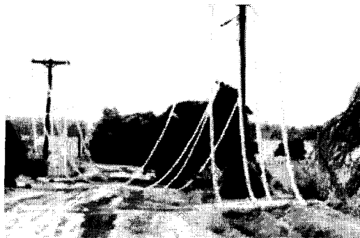
Figure 1.1. Wires collapsed under weight of ice accumulation.
