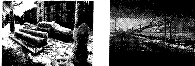
Figure 2.1. Icing (left); and destruction of power transmission line post and pylon caused by accumulated ice (right). (Ice Storm, Québec, January 1998.) [6, 28].
