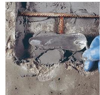
Figure 4.20 : Application du mortier
