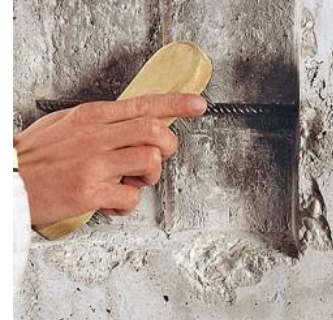
Figure 4.17: Elimination de la rouille
