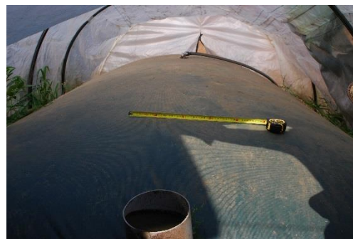
Figure 2: internal view of plastic bag digester.
