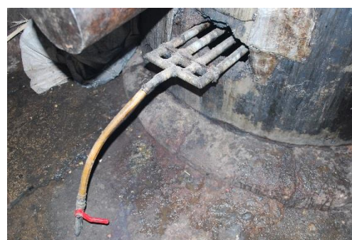
Figure 4: gas inlet for the 400 L cooker.
