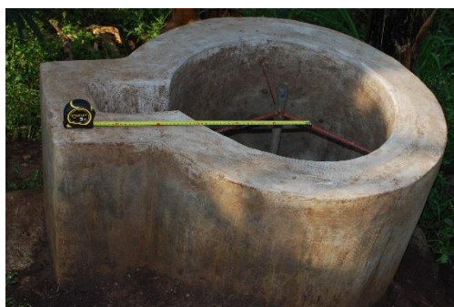
Figure 1: feed chamber, including scale (50cm).
