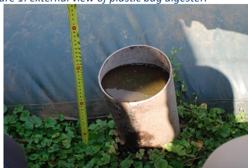
Figure 3: feed entrance, where mixing chamber should be added.
