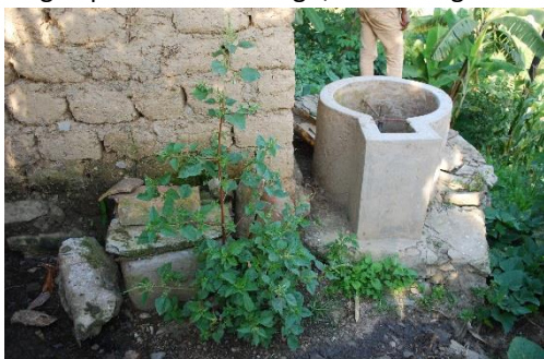
Figure 1: feed chamber (for cow dung) (right) and entrance for human waste to the digestion chamber (left).
