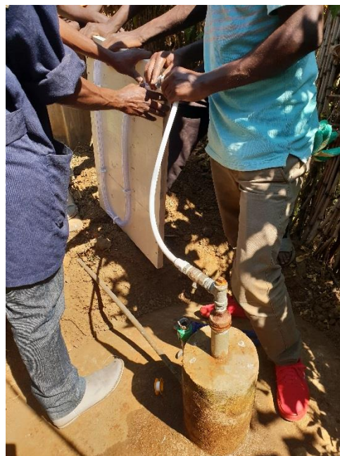
Figure 3: intern pressure check using a U manometer on the dome outlet valve.
