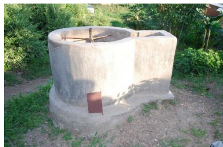
Figure 2: feed chamber, where cow dung is stirred.
