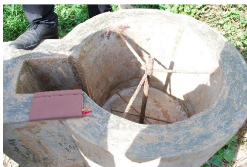
Figure 1 : feed chamber, where feed is added 4x a week.
