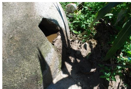
Figure 2 : slurry exit, moved by natural convection and reused as fertilizer.
