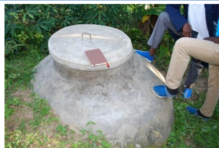
Figure 3: closed evacuation chamber.
