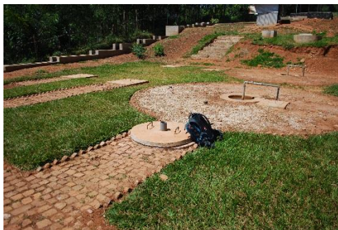
Figure 2 : 2x100m 3 digesters, built during phase 2 of construction and reserved for women waste.
