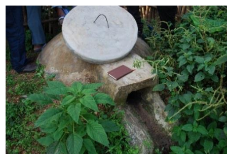
Figure 3 : evacuation chamber's exit, where slurry surplus is emptied and reused as fertilizer.
