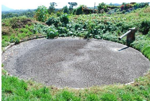
Figure 3: retention pond, containing slurry evacuated from 4x100m 3 digester (diameter 7m, depth 1.5m).
