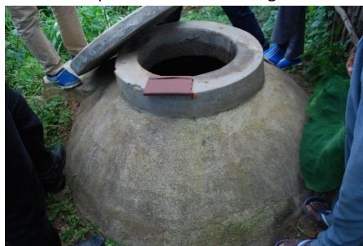
Figure 2: evacuation chamber, where measured temperature reaches 22°C.
