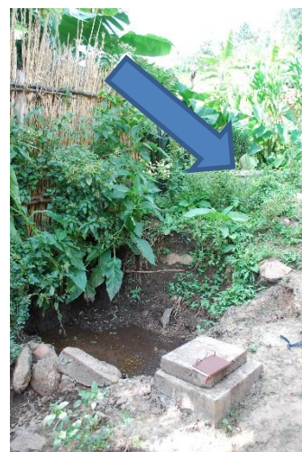
Figure 2 : digester chamber (blue arrow) and evacuation chamber (middle left). In the foreground, gas tap chamber.
