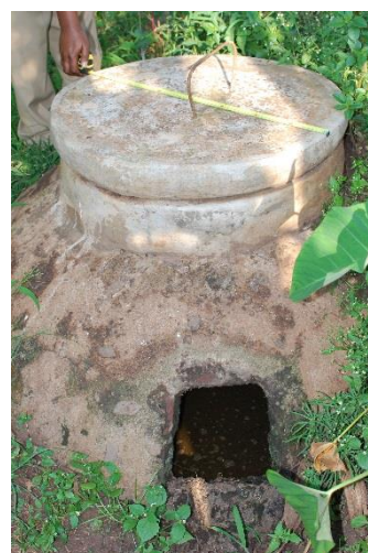
Figure 2: evacuation chamber, including scale (70cm).
