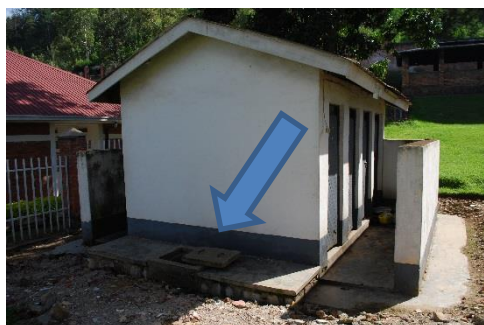
Figure 1: latrine, including human waste collector (blue arrow)
