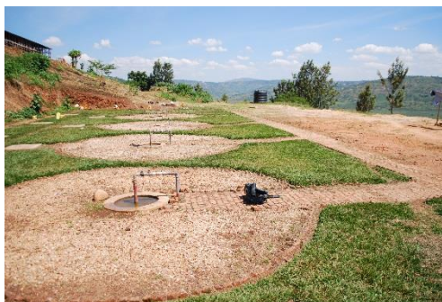
Figure 1 : 4x100m 3 digesters, built during phase 1 of construction.
