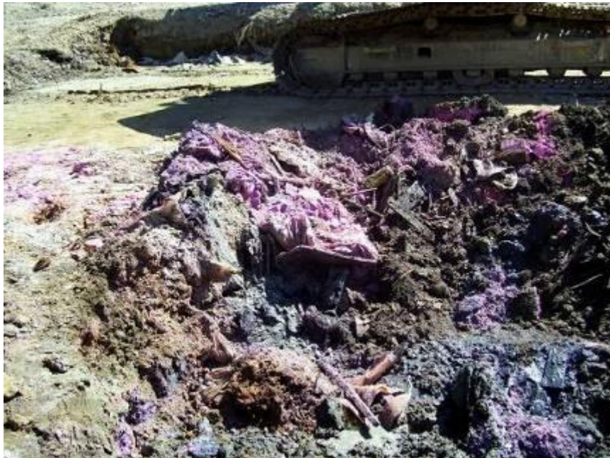
Figure 8. An example of in situ contaminated soil, dye, pure product, and debris
