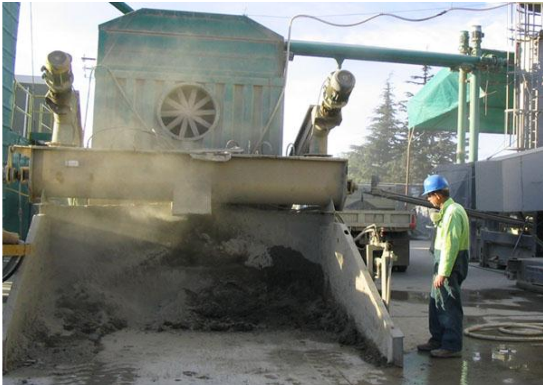
Figure 3. An EDL worker, with PPE but not wearing it, at exit from the reactors
