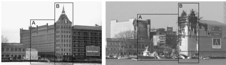
Fig. 1. Molino Stucky in Venice before and after the fire accident (A—collapsed wing and B—tower). (2003)
