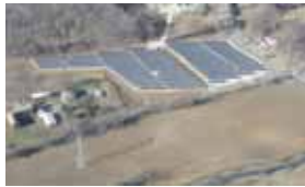
Source photo : PV Tech (1,6 MW Masonic Home of New Jersey, 5 656 modules K205)
