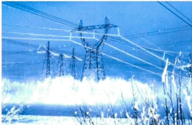
Figure 1.2 Snow accumulations on transmission lines during New Jersey storm 2011 (Snow Murray web site).
