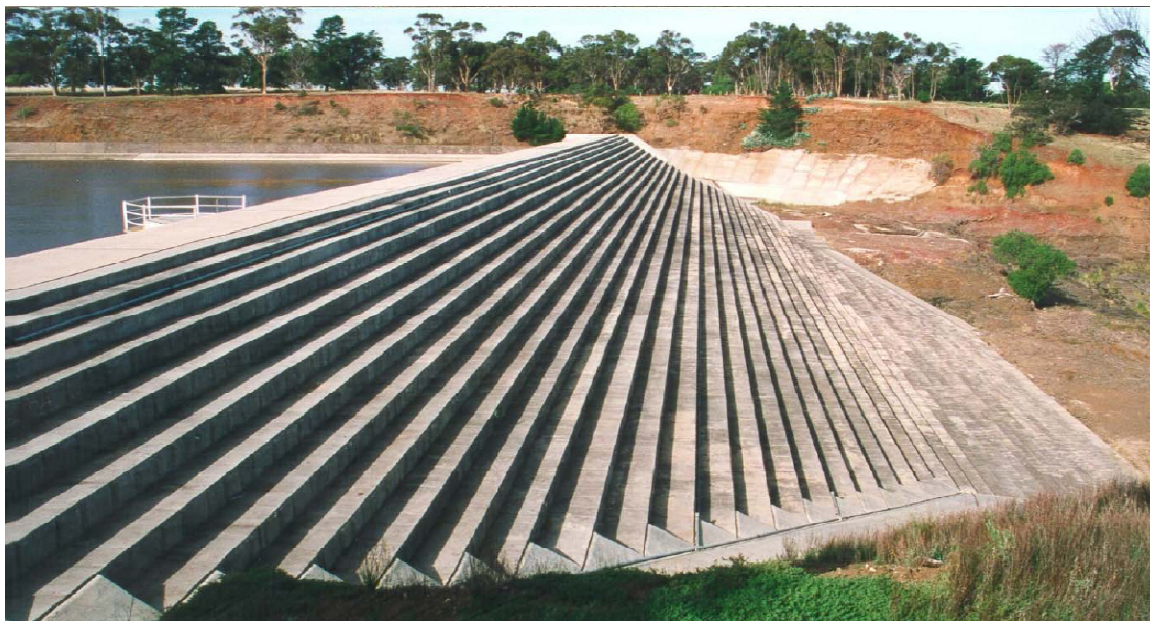
B: Melton dam secondary spillway (Australia)
