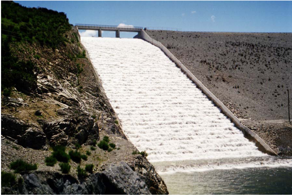
A: Stepped spillway of the Opuha embankment dam
