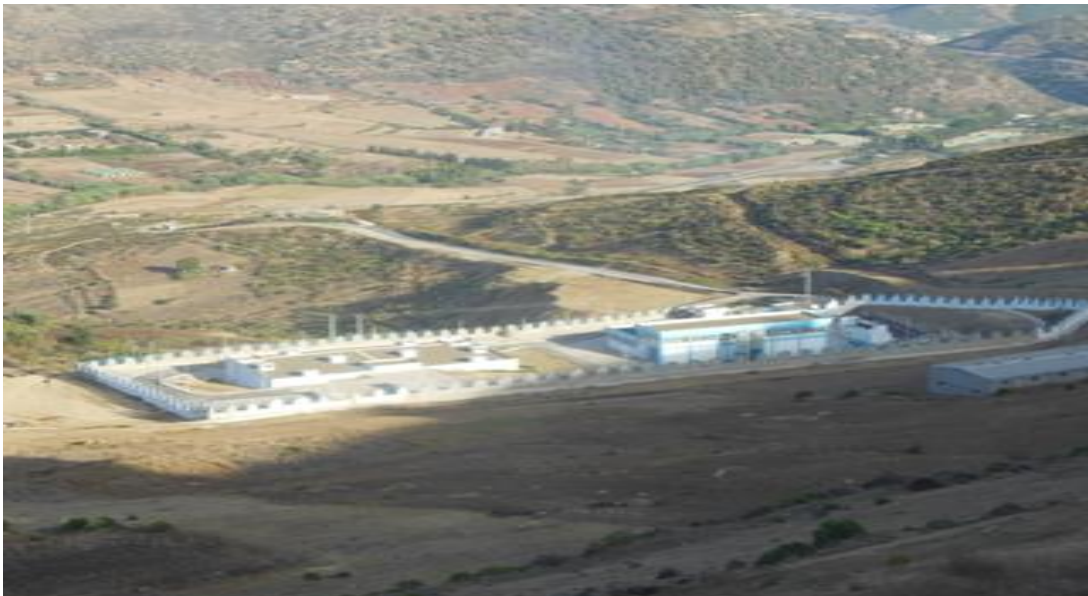
Photo II.3 Station de pompage HSP1 [27]
