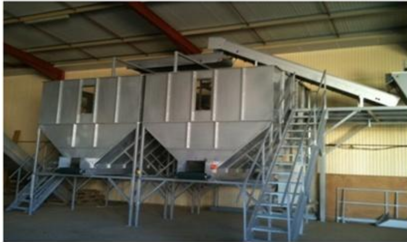
Figure 3.3 : trémie de stockage plants. [34]
