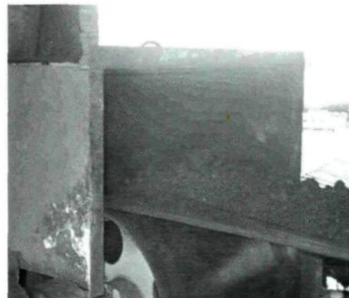
Figure 4.4 Coke conveyor and feeding hole
