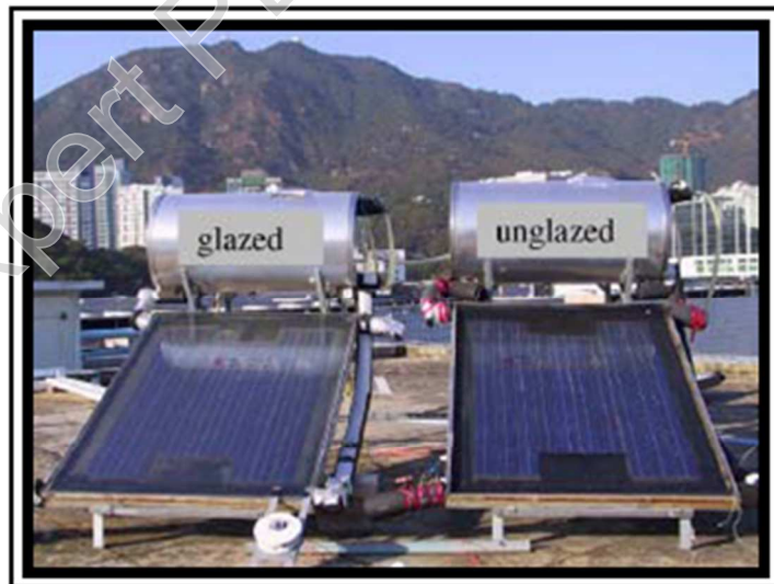
Figure 3-16: Premier et second prototypes construits [45]
